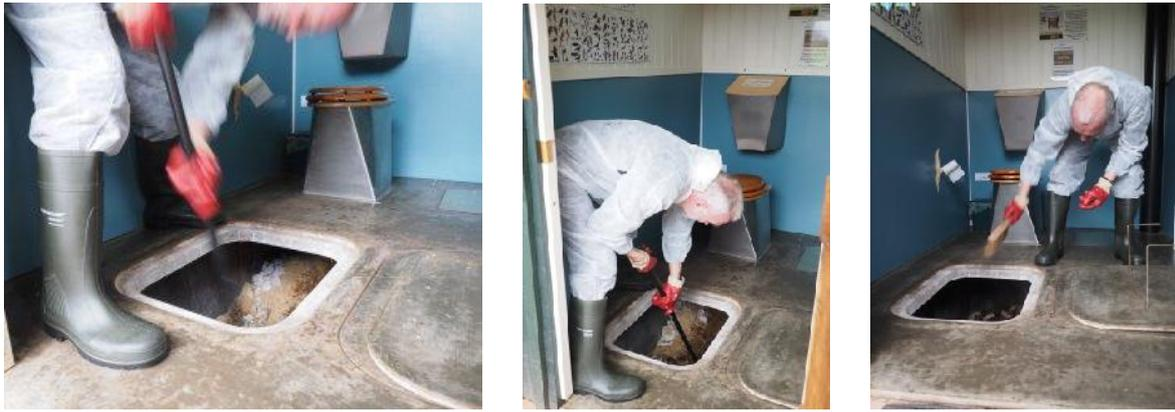
Raking the compost towards the door end and sweeping the flange before refitting the hatch.
