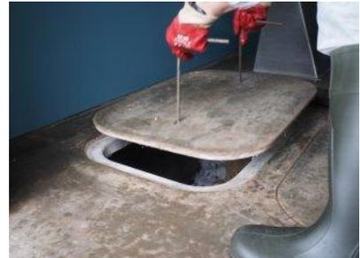
Check the compost pile for “peaking” and if required use the rake **stored in this vault** to bring the pile towards the front (door) end of the vault. This prevents excessive build up of compost directly below the toilet which could ultimately impede the function of the urine gutter. At no time should the compost be closer to the urine gutter than about 100mm. This operation also helps to bring the pile into the final position for emptying after the vault resting period.
